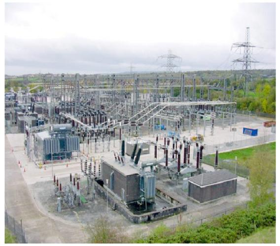
Figure 4.3: Air Insulated Substation (Source: http://www.foxitsoftware.com)
